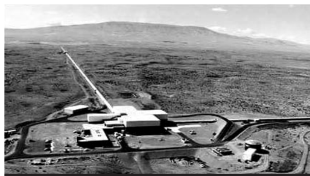
The LIGO facility in Hanford, Washington, showing the two beam tubes, each four kilometers long.
