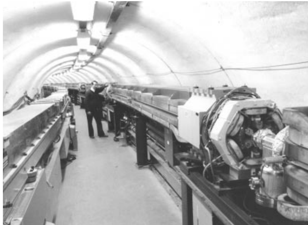
This tunnel under Robison Alumni Fields houses the Cornell Electron Storage Ring (CESR). The arc on the left, called a synchrotron, ramps the electron and anti-electron beams to the needed energy. The beams are then transferred to CESR itself, on the right, where they circulate, colliding once per revolution in the heart of our particle detector, CLEO. After one hour of collisions, the beams are noticeably depleted, and we restock them once again. Nearby, the Cornell High Energy Synchrotron Source (CHESS) takes advantage of x-rays produced by the beams to do a variety of research, including materials science, geophysics, and biology.
